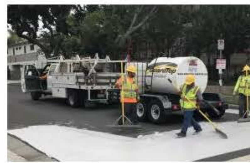
The city of Los Angeles is coating streets in a special gray paint that can lower the temperature as much as 10 degrees. (City of Los Angeles)
